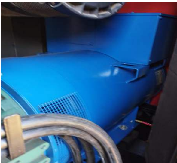
Installation of a new alternator on the standby Generator at Biggarsberg WPP
