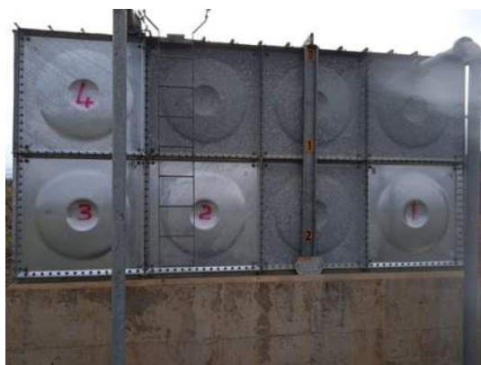
Replacement of panels on the storage tank at the Alcockspruit pump station
