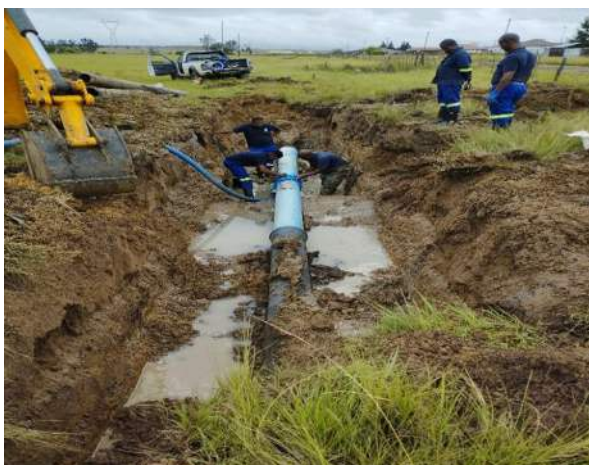
Repairing a burst on the Ngagane pipeline
