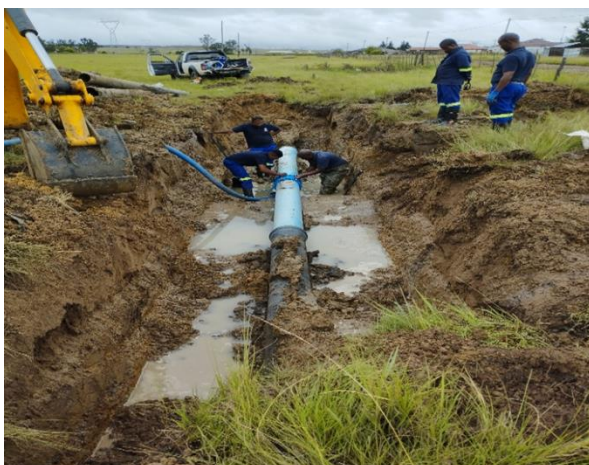
Repairing a burst on the Ngagane pipeline
