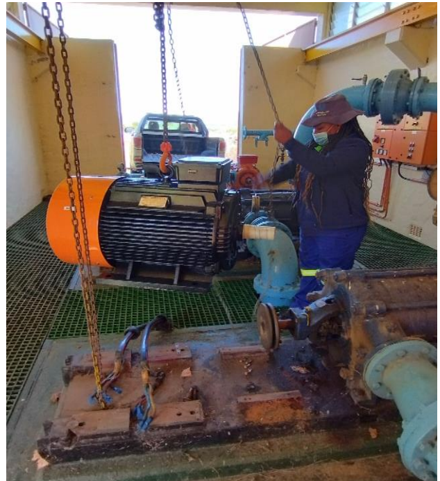
Figure 25: Installation of a new electrical motor at the Glencoe pump station.
