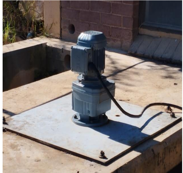
Figure 27: Installation of a new mixer at the Biggarsberg Water Purification Plant.
