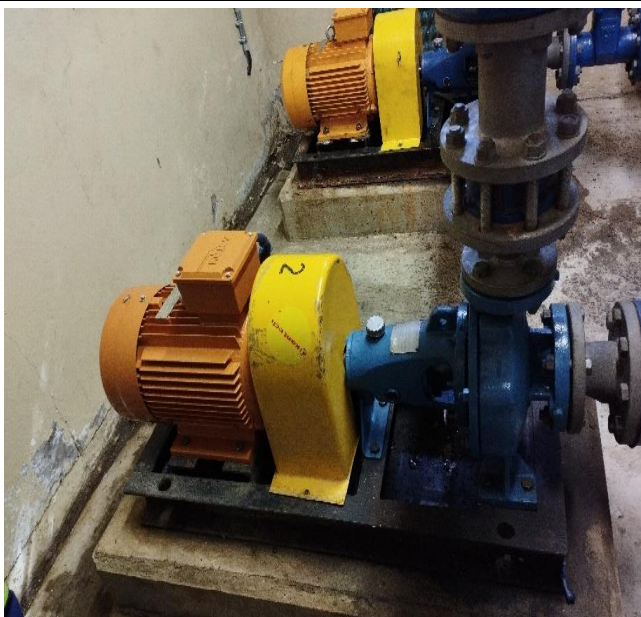
Figure 28: Installed a new electrical motor at the Indian village pump station.
