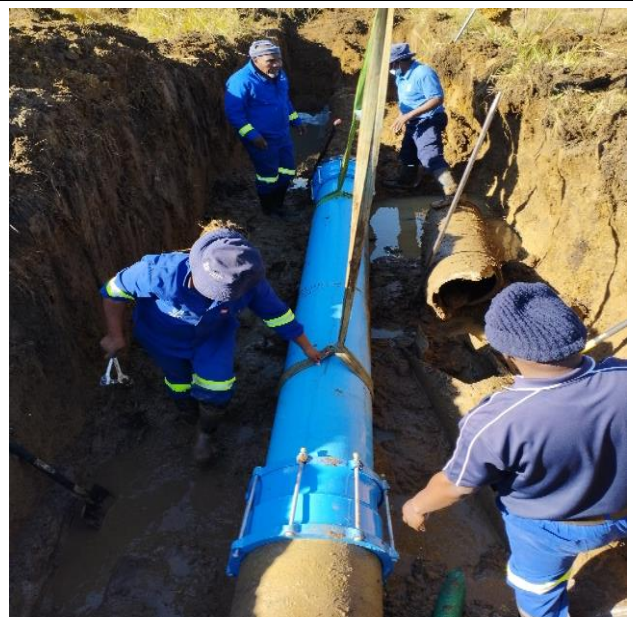
Figure 29: Repair of a burst on the Verdruk raw water pipeline.
