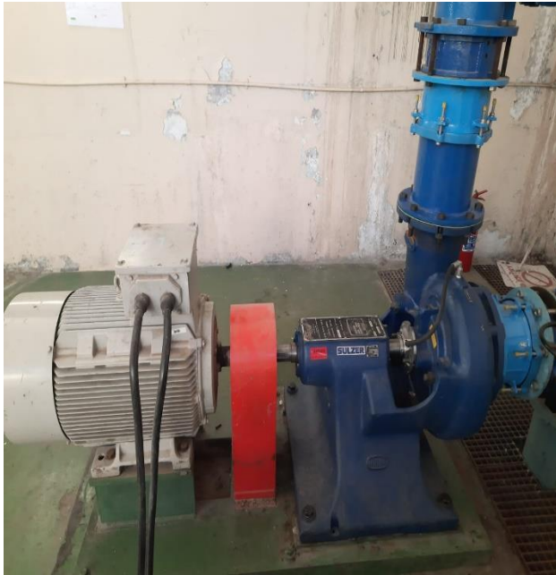
Figure 26: Installation of a new mechanical seal on the Backwash pump at the Ngagane Water Purification Plant.
