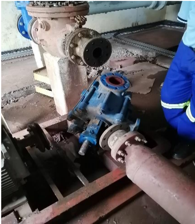
Figure 18: Removal of a faulty multi-stage pump at the Verdruk pump station.
