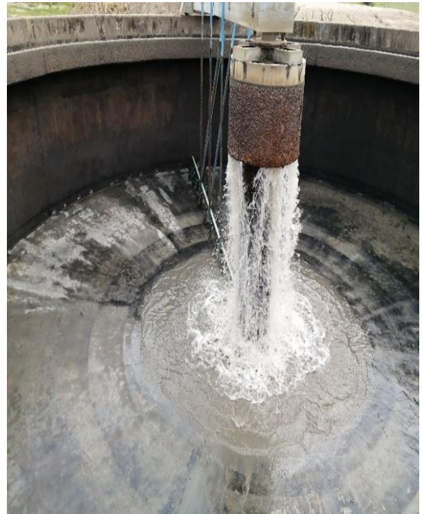
Figure 19: Refilling the Clarifier after cleaning at the Tayside high lift pump station.
