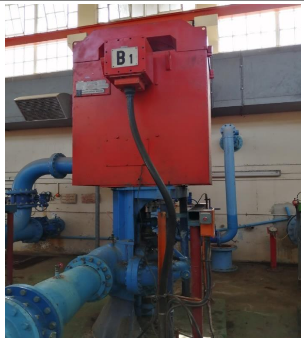
Figure 21: Removal of an electrical motor for testing at the Ngagane WPP.
