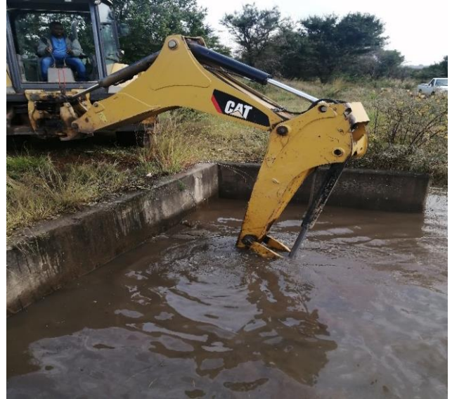
Figure 23: Cleaning the inlet chamber at the Buffalo river weir.
