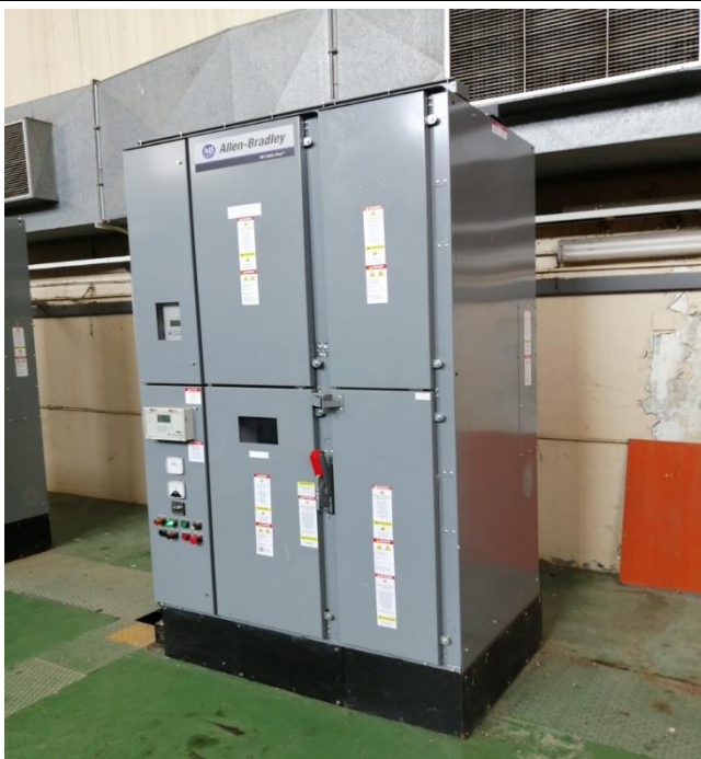
Figure 20: Tracing an electrical fault incurred on the A-Pump panel at the Ngagane WPP.
