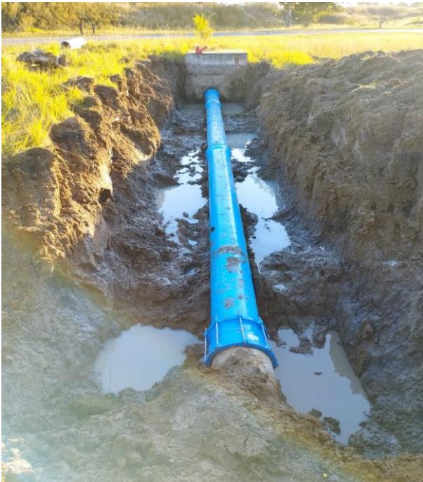
Figure 24: Repairing a burst on the Hilldrop AC pipeline
