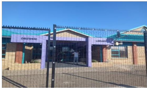
Figure 23 New fencing erected at the Osizweni Library
