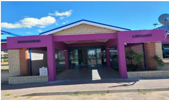
Figure 22 Renovated Madadeni Library
