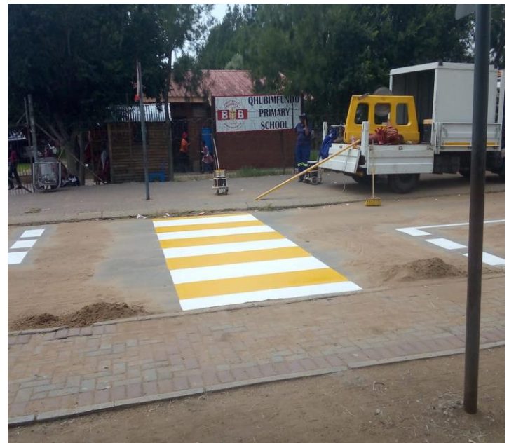
Pedestrian crossing marking and road warning sign installation
