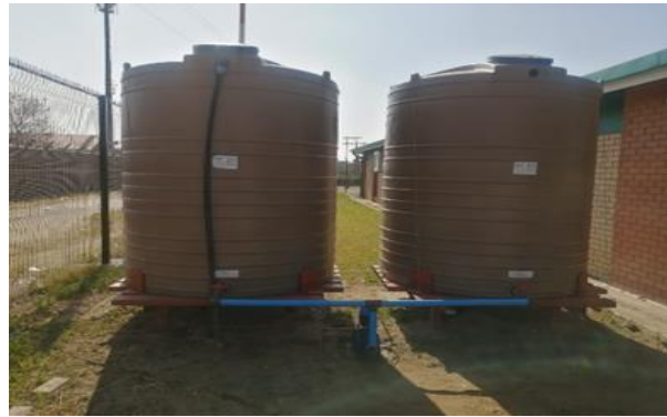
Figure 21 Borehole at Osizweni Library
