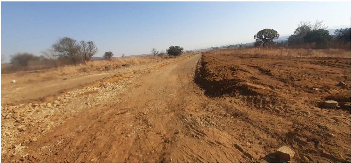
Hastie Street Site progress
