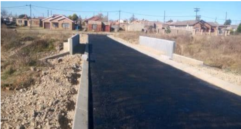
UPGRADE OF MF7, MF10 AND MF69 ROADS
