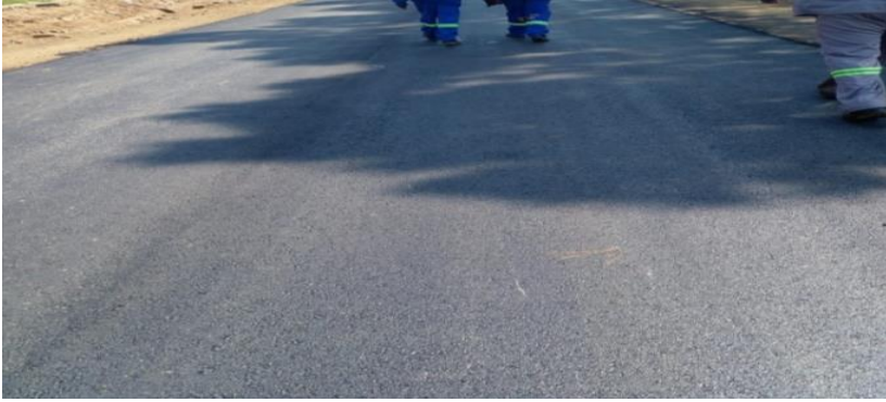
UPGRADING OF MF18 AND MF19 TO BLACKTOP IN MADADENI
