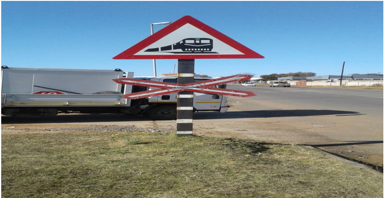
Installation of road warning sign for railway crossing lane
