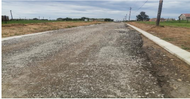
CONSTRUCTION OF OB1 LINK ROAD
