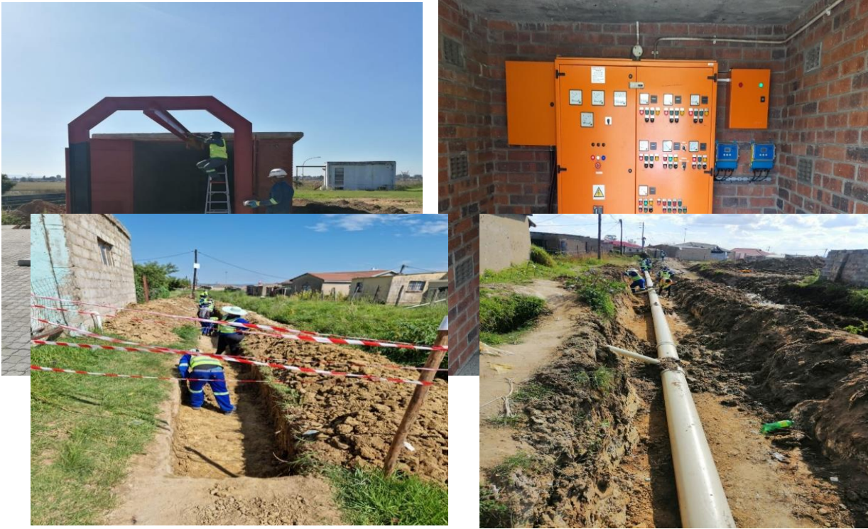
REPLACEMENT OF THE DN150 BULK OUTFALL SEWER CLAY PIPELINE IN STAFFORDHILL
