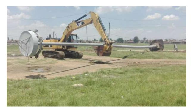
Figure 13 INSTALLATION OF A HIGH MAST LIGHT
