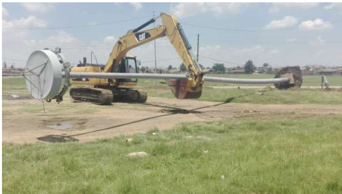
Figure 13 INSTALLATION OF A HIGH MAST LIGHT
