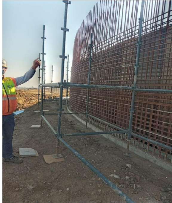
Reinforcing steelwork for reservoir walls
