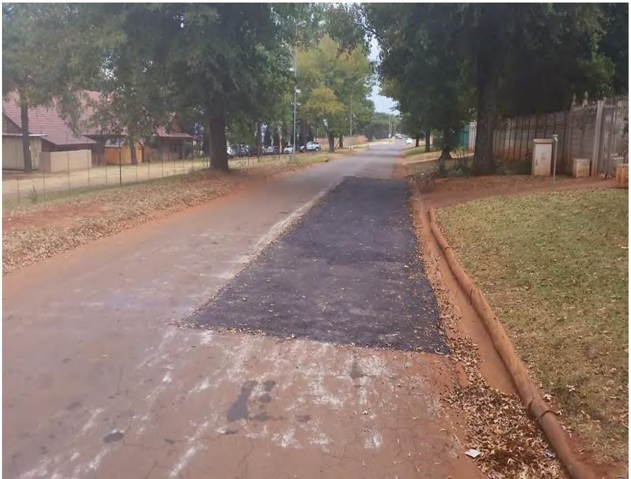
Figure 63 tar patching at aquamarine drive
