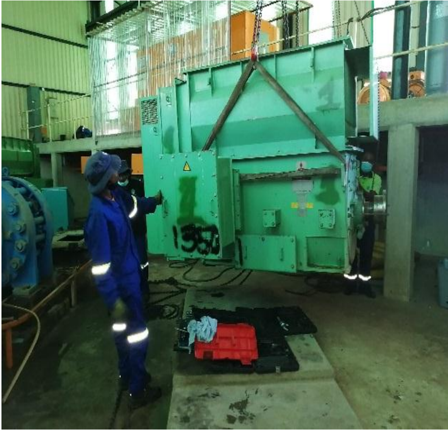
Removal of the Electrical motor repair Tayside high lift pump no.2
