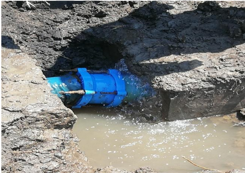
Repairing a coupling on Kilbarchan pipeline to the reservoirs
