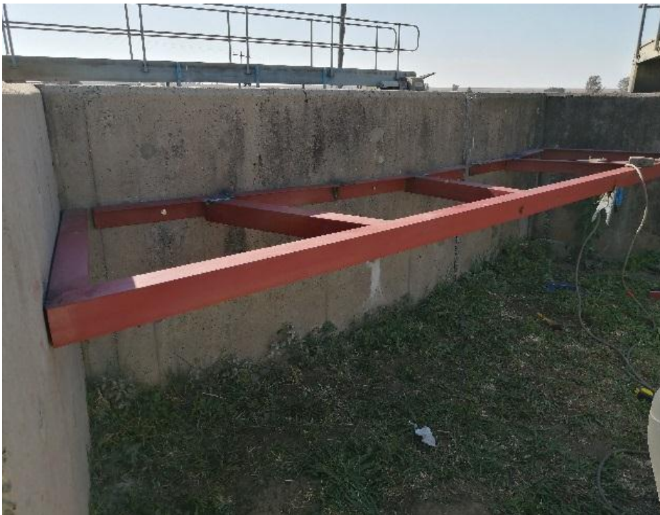
Fabrication of a platform for the Clarifier at Tayside pump station
