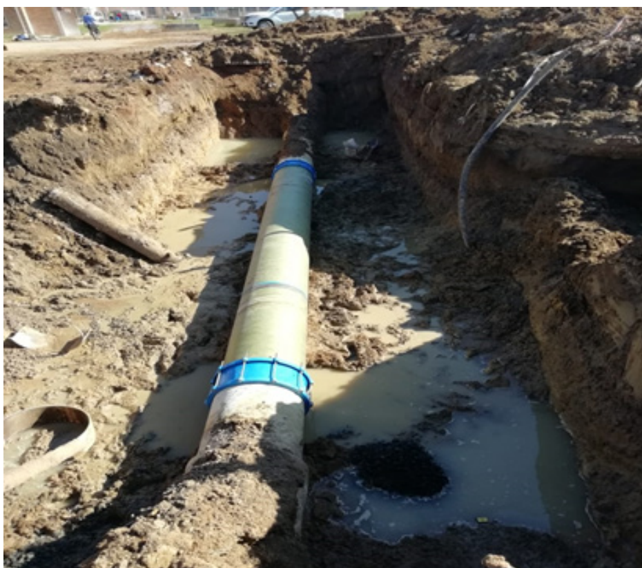
Repairing of the GRP Pipeline from the Ngagane Water plant to Braakfontein reservoirs
