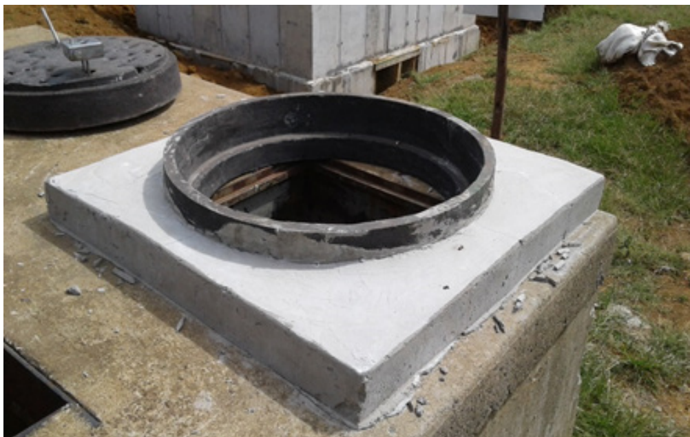
Installation of a new lockable lid for a valve chamber on the Ntshingwayo raw water pipeline
