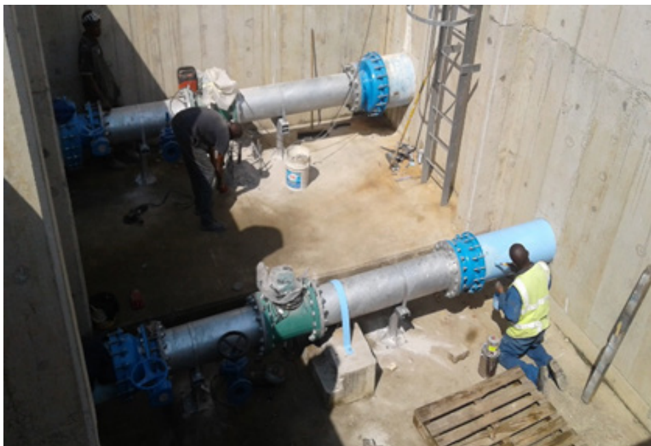
Installation of new electronic flow meters at the Ngagane Water Purification Plant
