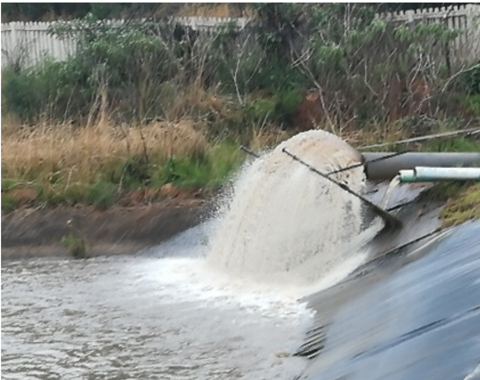
Pigging of the Tayside raw water pipeline.
