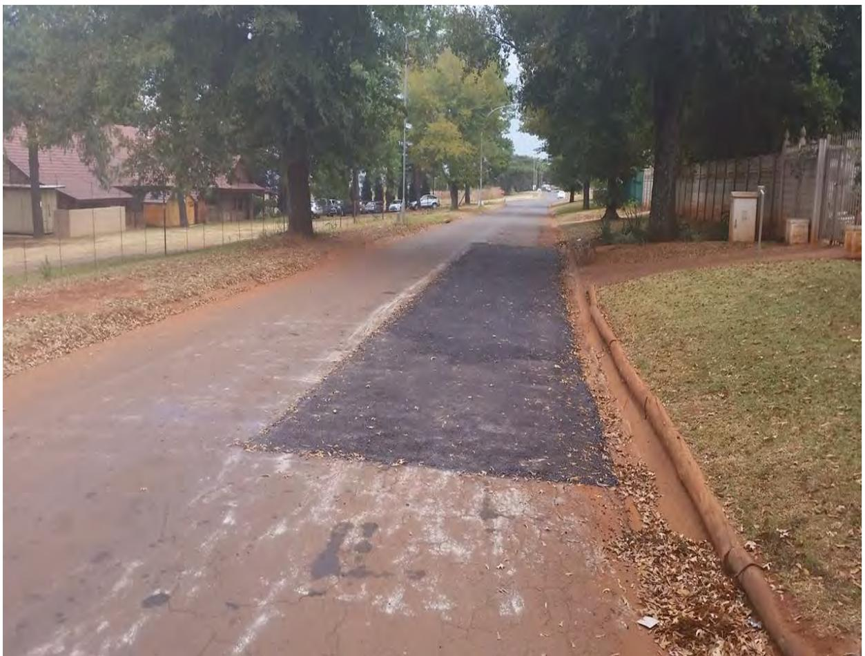
Figure 63 tar patching at aquamarine drive
