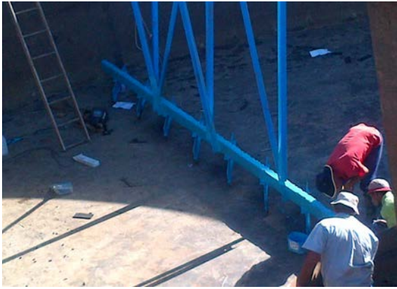
Clarifier bridge repair
