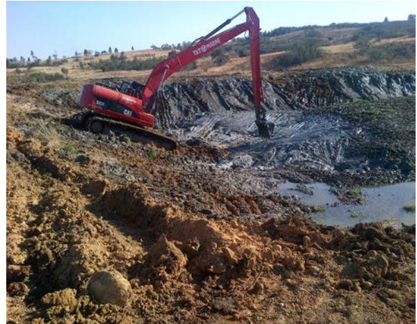
De-sludge of the sludge dam below the sludge drying beds.
