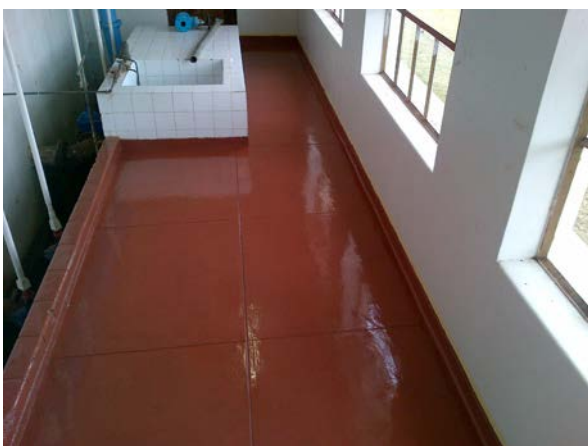
Civil repairs and painting of the filter clear water plant section.
