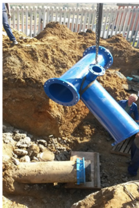
Replacement of a pipeline section on the Tayside pipeline.
