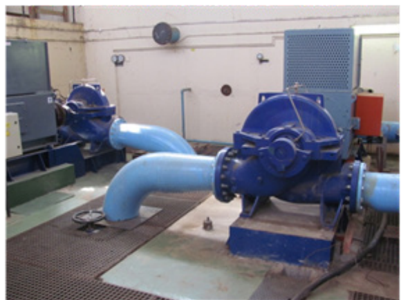
New installation of the D-Pumps and reconditioned B-pump.
