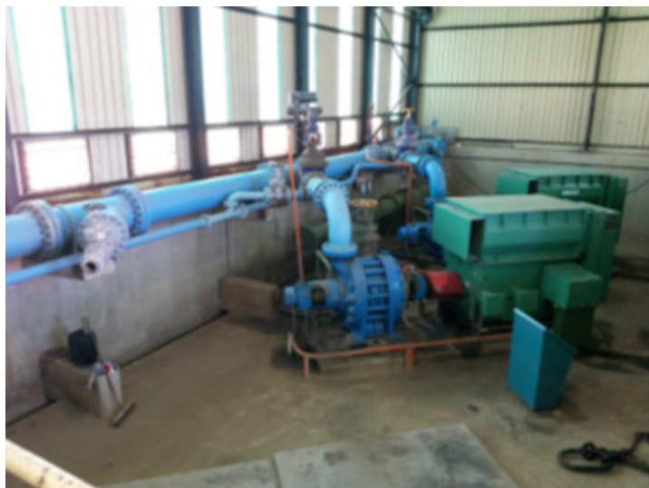
Tayside high lift pump station
