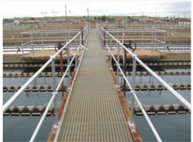
Replacement of the hand rails at the filters to ensure that safety regulations are adhered to.
