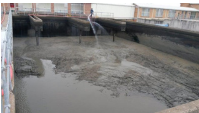
Cleaning of Plant 2 sedimentation tank.
