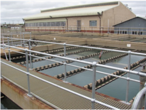
Replacement of the hand rails at the filters to ensure that safety regulations are adhered to.
