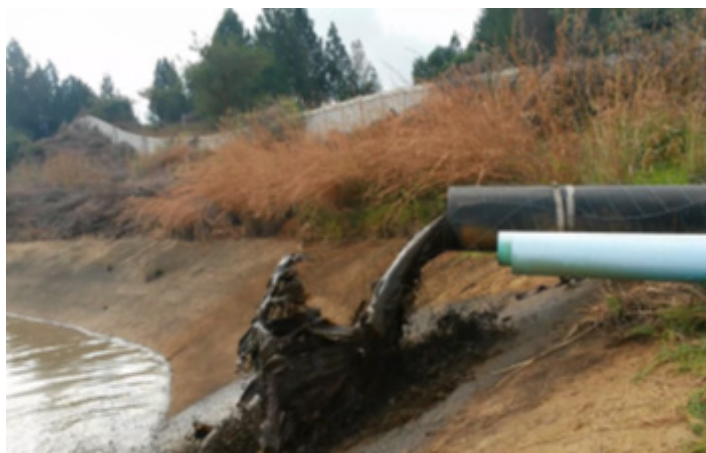
The exit of the last pig resulted in removing debris on the inside of the pipeline
