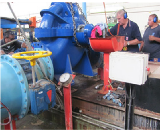
Installation of a new Split Casing Pump at the Ngagane Plant main pump station.
