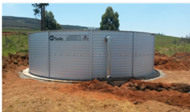
Steel 100 Kl steel tank and pipeline laying
